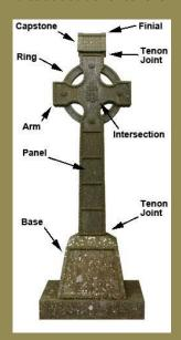
The major components of the Celtic, or high cross are the cross base, intersection, ring, and capstone (including the finial). Construction of the Celtic cross normally starts with the cross base, which is an extremely heavy stone. Often times, the base had another life before being carved for the cross, such as being used as a millstone. The high cross is seated into a carved socket in the stone base by means of a tenon, forming a very secure and strong joint.
