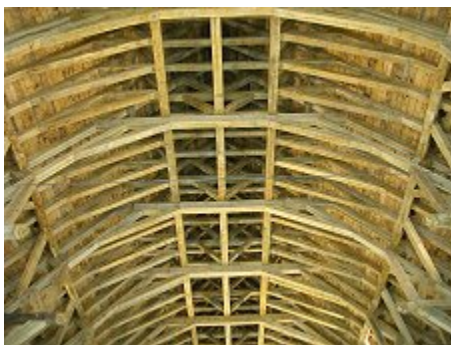
Hammerbeam vaulted roof
